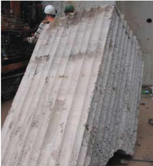
The concrete slab stretched to 2 metres in depth in places.
